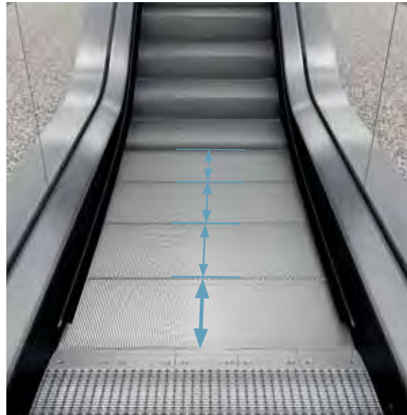
Figure 5.10 Horizontal steps enable a passenger to step safely on and off the escalator.
