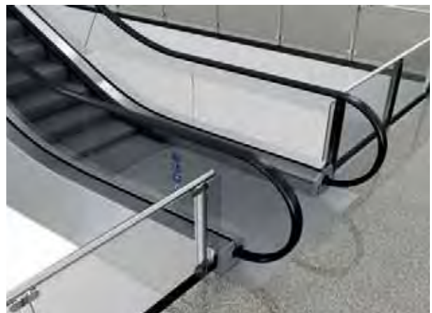
Figure 5.19 An extended balustrade allows railings to neatly butt against the escalator balustrade
