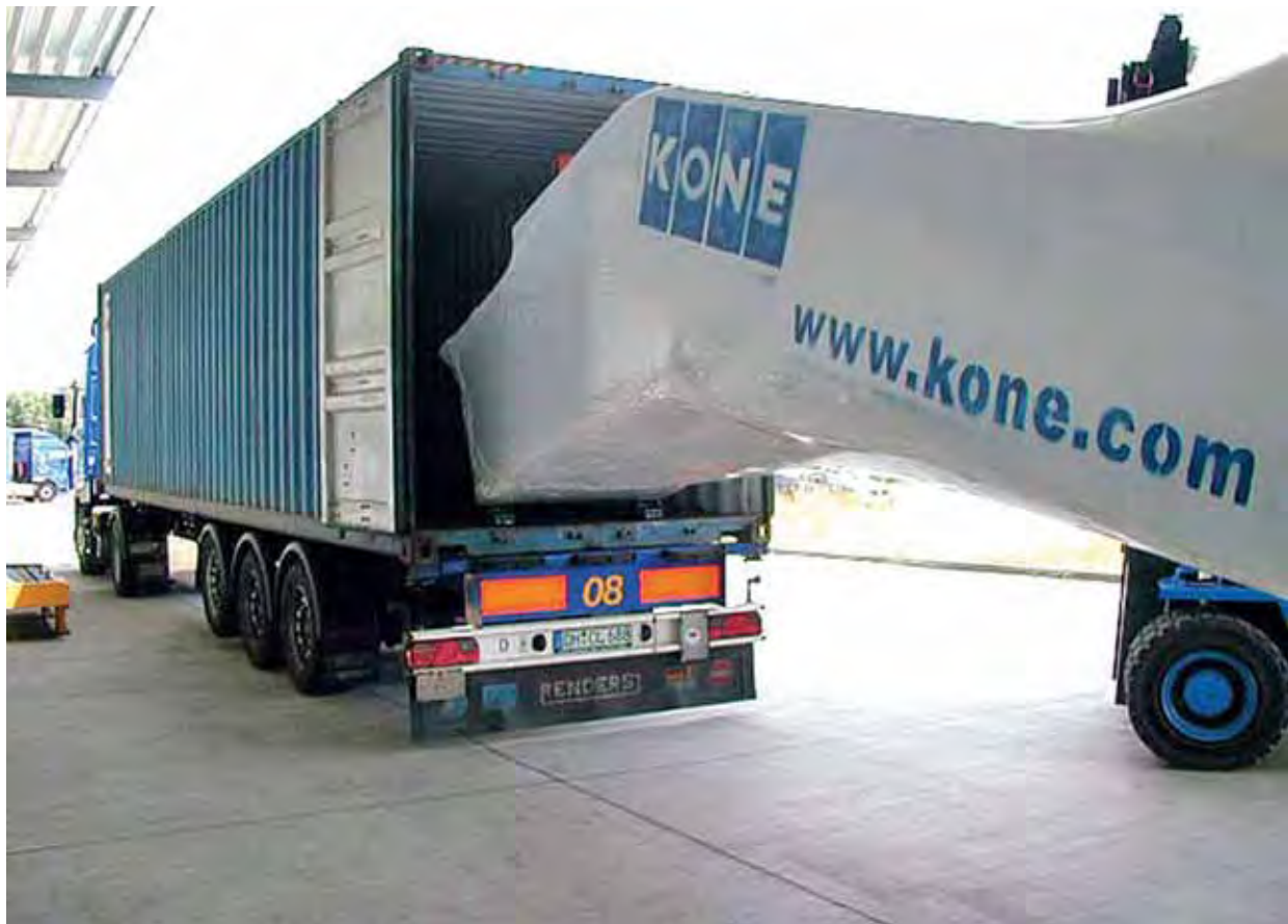
Figure 7.7 Unloading an escalator using forklift trucks
