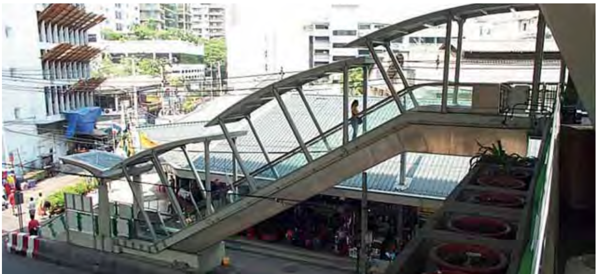
Figure 4.3 The outdoor escalator should be covered by a roof to improve passenger safety and convenience.
